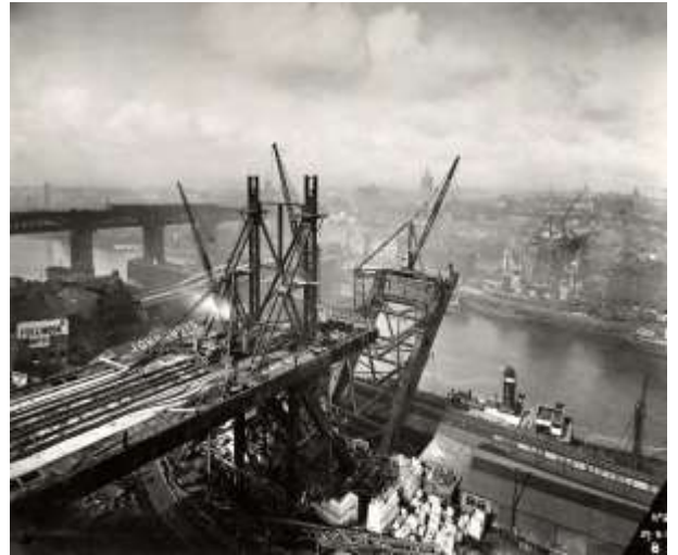
Dorman Long Collection - Building the Tyne Bridge, 1927, Courtesy of AmberSide Collection
